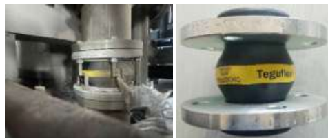
Expansion Joint used in Slurry pipeline
